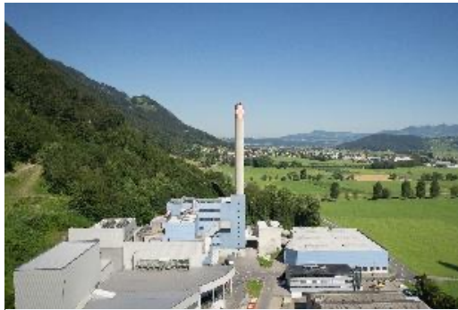
KVA Linth, Switzerland
